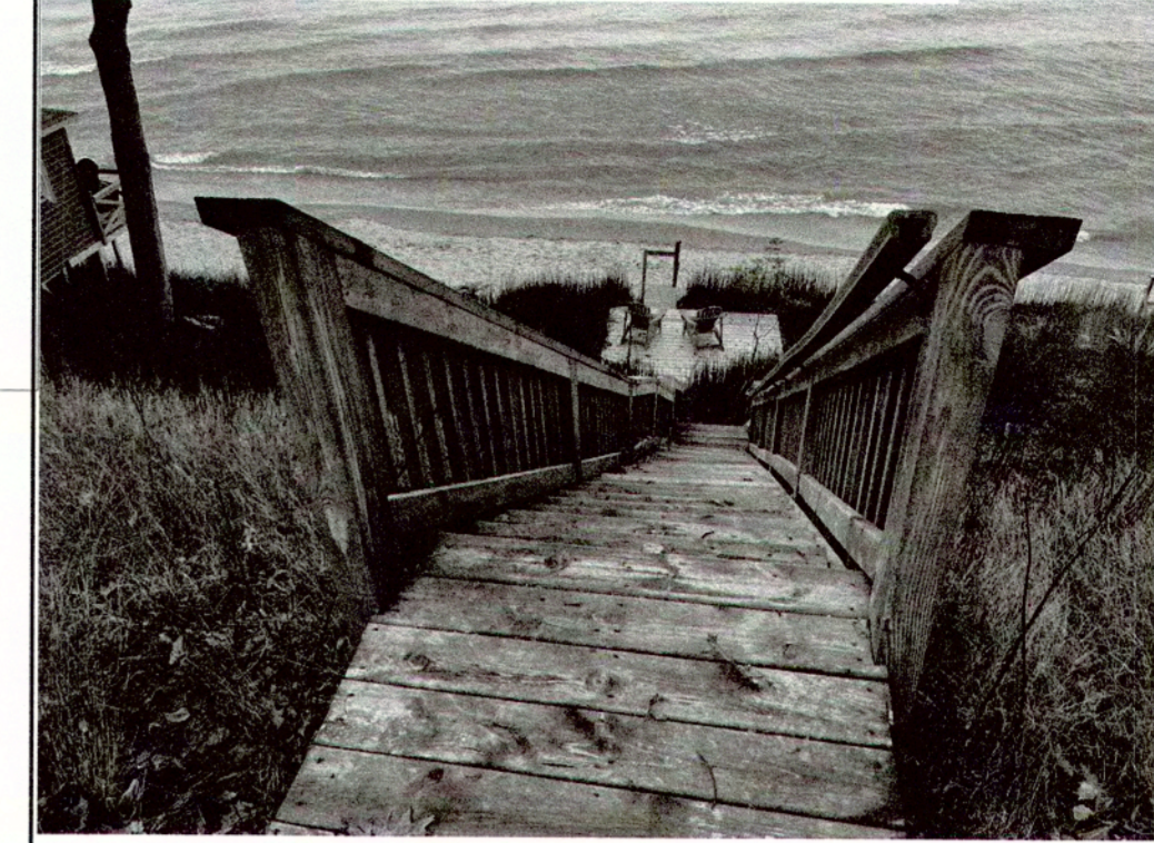
VIEW OF STAIR TO BE REPLACED
